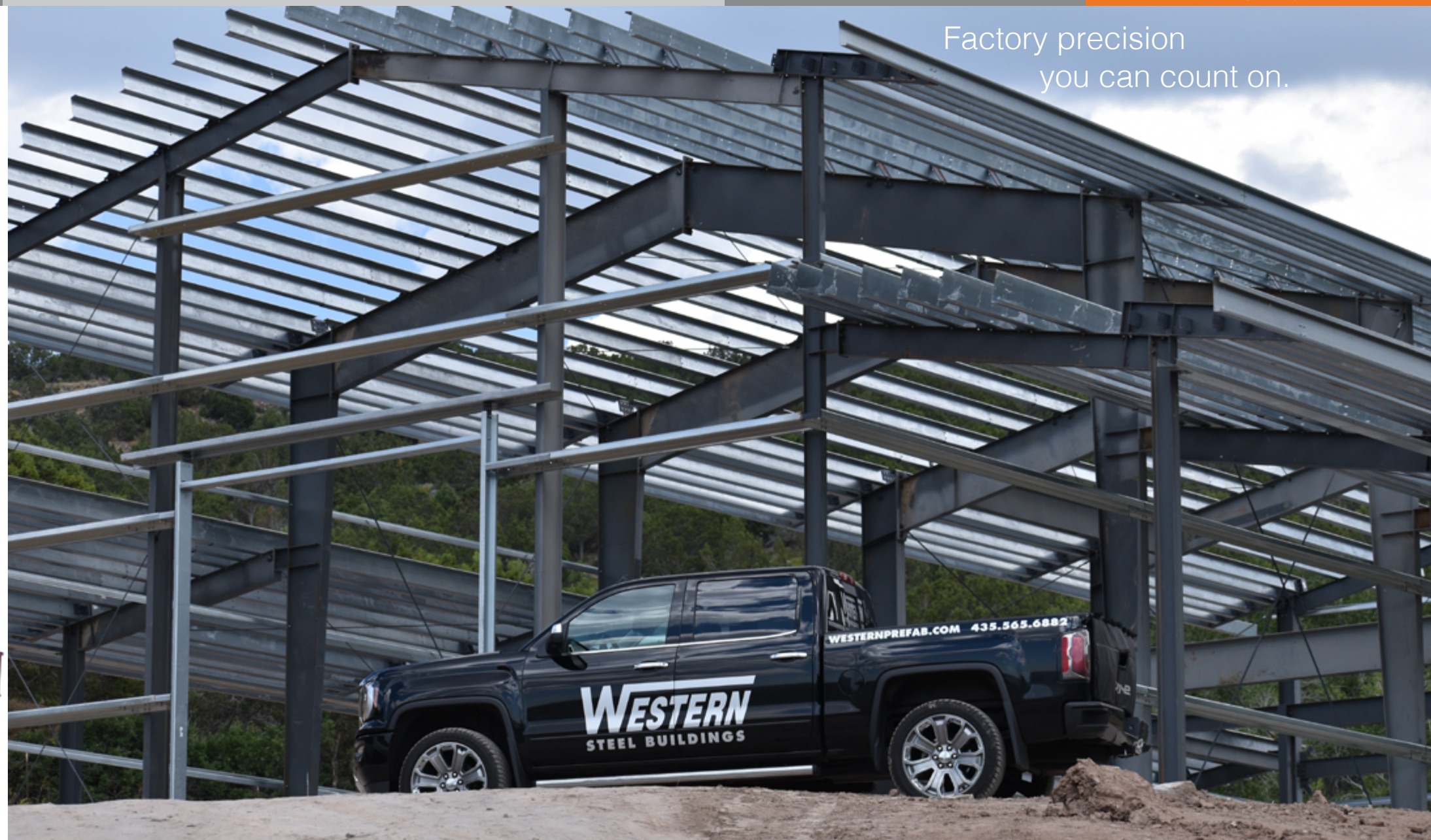
42'0" x 80'0" x 20'0" with 13'0" Sidewall Lean-to Frames Double Slope, Clear Span Building, Lean-To on SWA & SWC Straight Frames (shown in image to the right)
